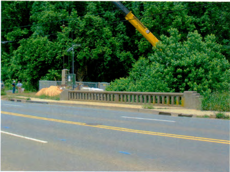
No. 20 Stewart Creek Bridge.
