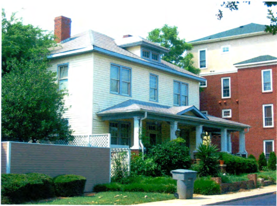
No. 9 House, 328 South Cedar Street.
