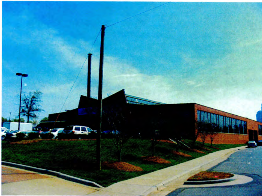
No. 16 West Morehead Street Industrial Historic District, (Former) Grinnell Company Building.
