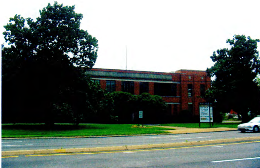
No. 30 General Dye Stuffs Corporation Building.
