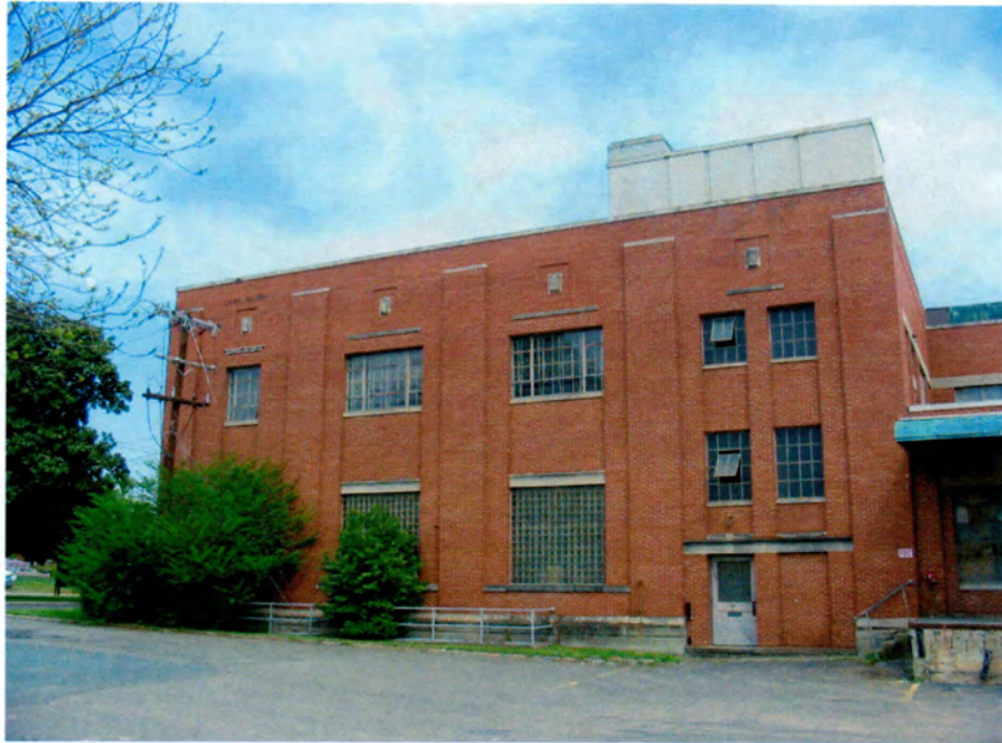
No. 30 General Dye Stuffs Corporation Building.
