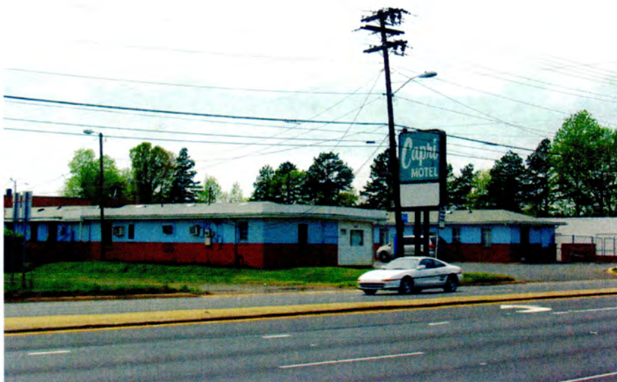
No. 41 Dixie Motor Court (Capri Motel).
