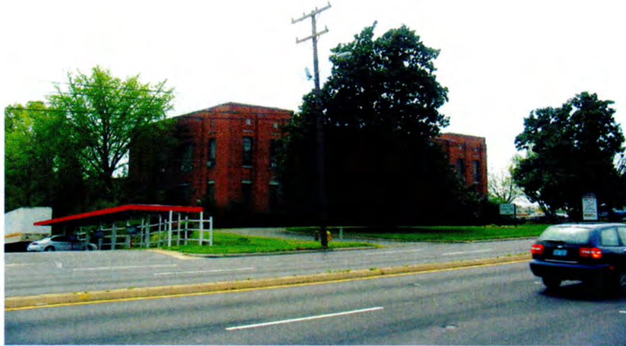
No. 30 General Dye Stuffs Corporation Building.
