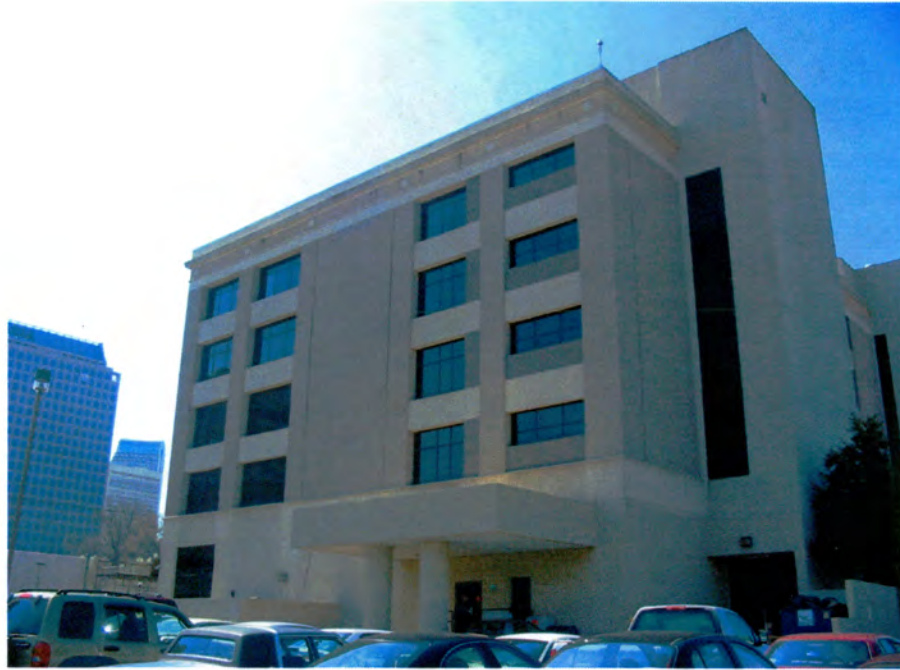
No. 5 Coddington Building (Polk Building), Rear Elevation.
